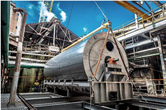
*CAPTION: The first mud filter is lowered onto its foundations inside the factory.*
