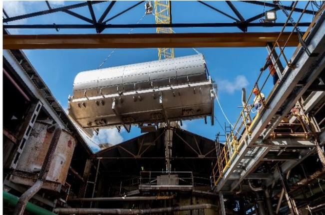
*CAPTION: A 400-tonne crane is used to lift the first of Victoria Mill's two new mud filters in through a temporary opening in the factory's roof.*
